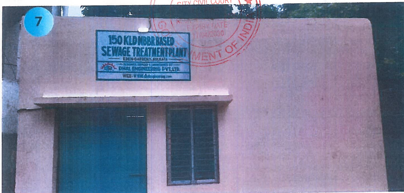
STP PLANT ROOM FRONT SIDE
