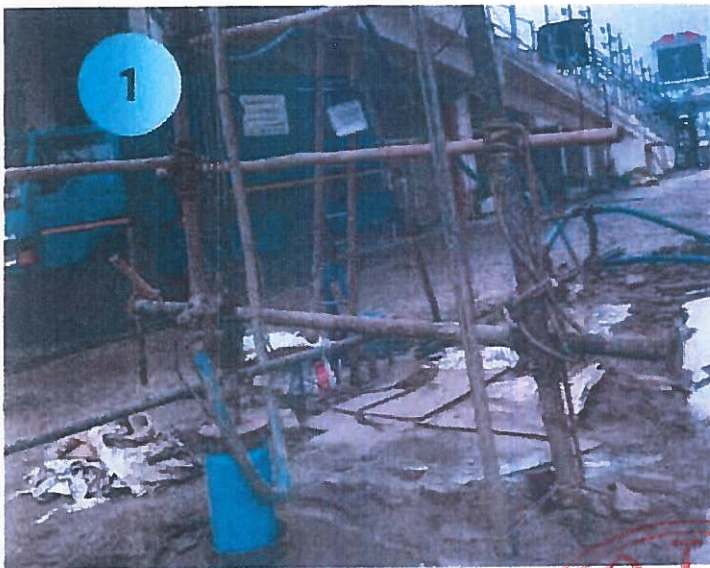
Completed Borewell at Location #1
