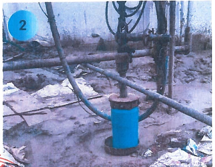
Completed Borewell at Location #2
